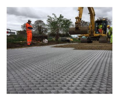
Geo textile, the high strength polypropylene is widely used to filter, stabilize, reinforce, separate, drains and isolates soils in categories of civil construction applications.
